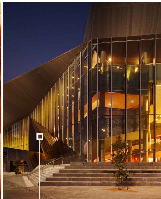
MELBOURNE EXHIBITION AND CONVENTION CENTRE WOODS BAGOT AND NH ARCHITECTURE (2009, 126000sq.m, $1B)
